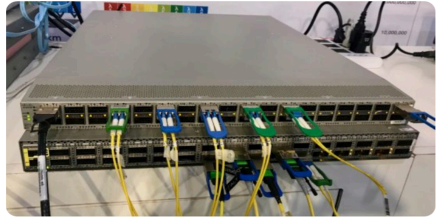
Cisco's Nexus 400 GbE (bottom) and 100 GbE 32 port switches in action in the demo
